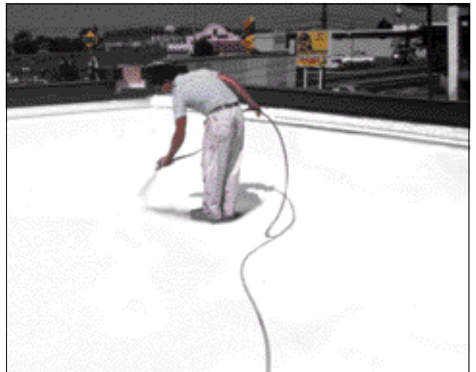
Step 4 TOPCOAT finish coat is applied
