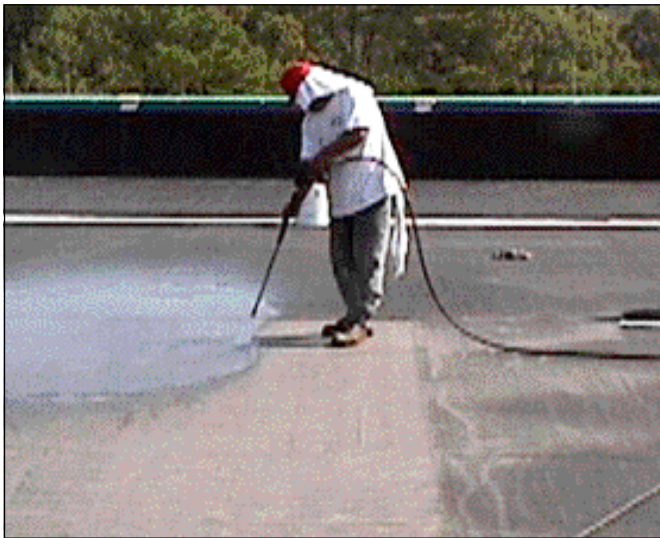
Step 1 Existing roof is thoroughly clean & repaired
