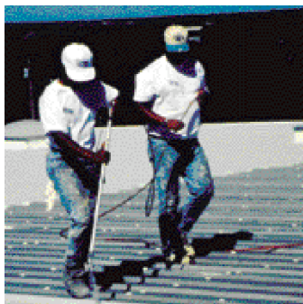
Step 10 TOPCOAT base coat is applied
