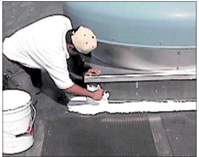
Step 2 All seams and protrusions are sealed
