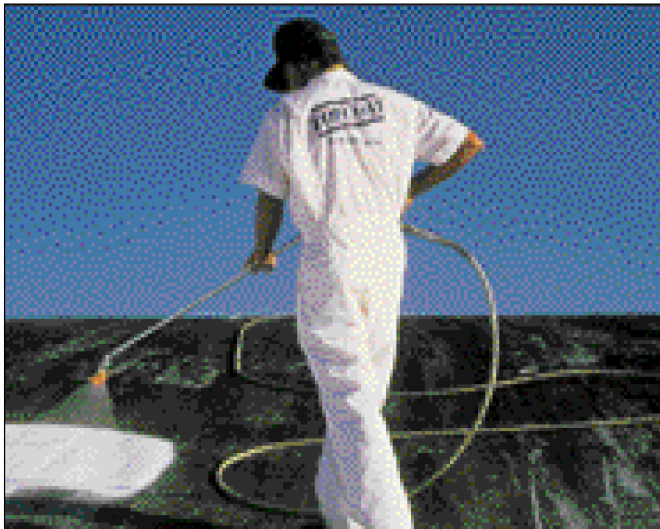
Step 3 TOPCOAT base coat is applied
