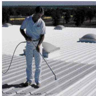
Step 11 TOPCOAT finish coat is applied
