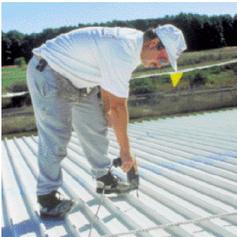
Step 1 Fasteners are tightened and/or replaced
