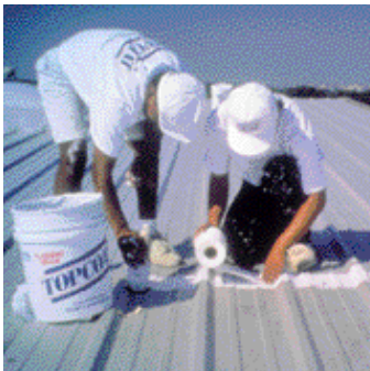
Step 5 Horizontal seams are sealed
